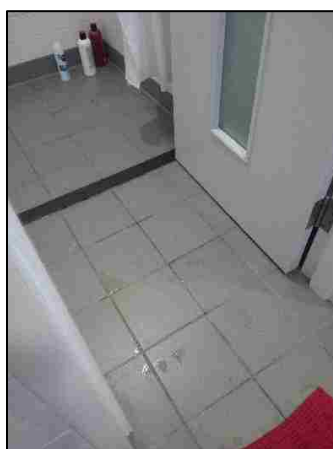
Figure 129: Shower sill in typical bathroom
