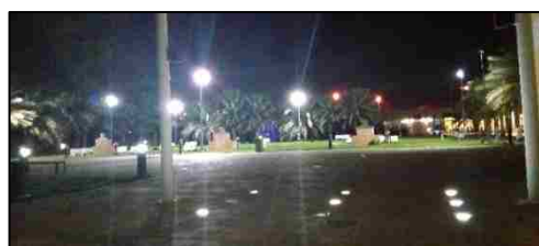
Figure 98: Lighting in the main garden
