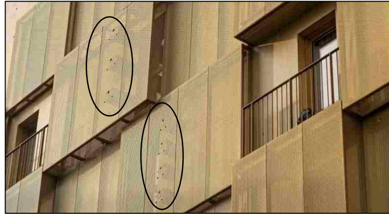
Figure 30: View of the birdhouses from the exterior façade of golden student housing in Paris – Source: (Gibson, 2016)
